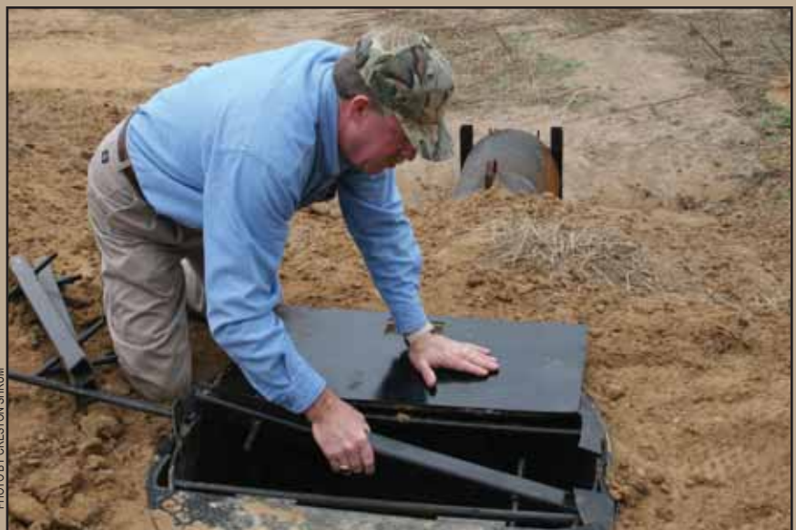
David Fowlkes inserts boards into a water control structure.
